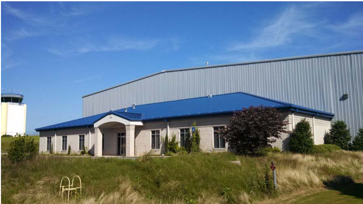
Front View of Office Area
