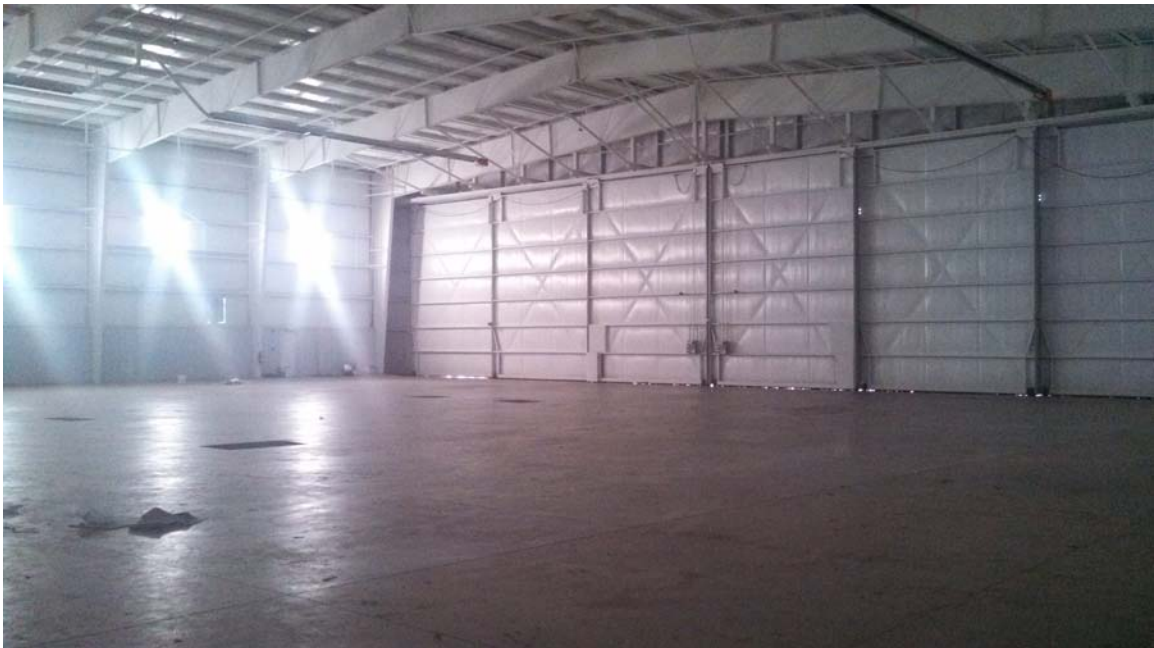
Interior Shot of Hangar
