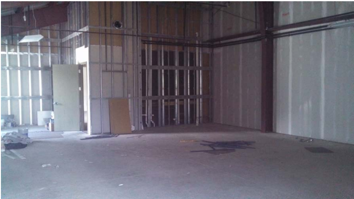
Unfinished Portion of Office Space
