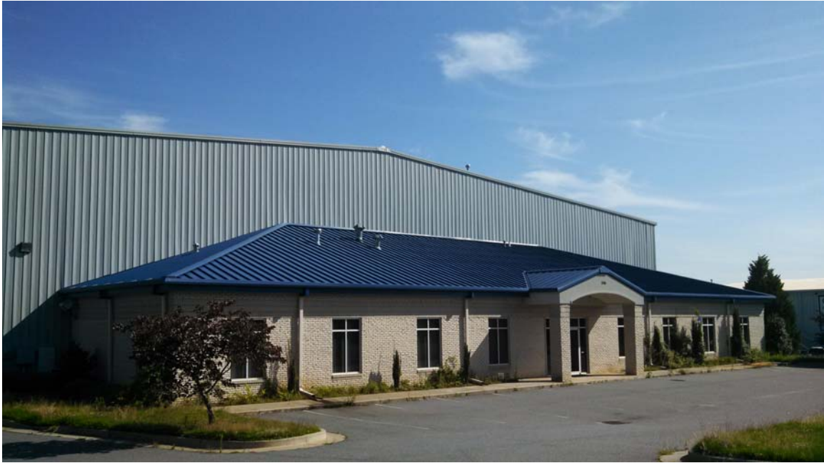
Front View of Office Area
