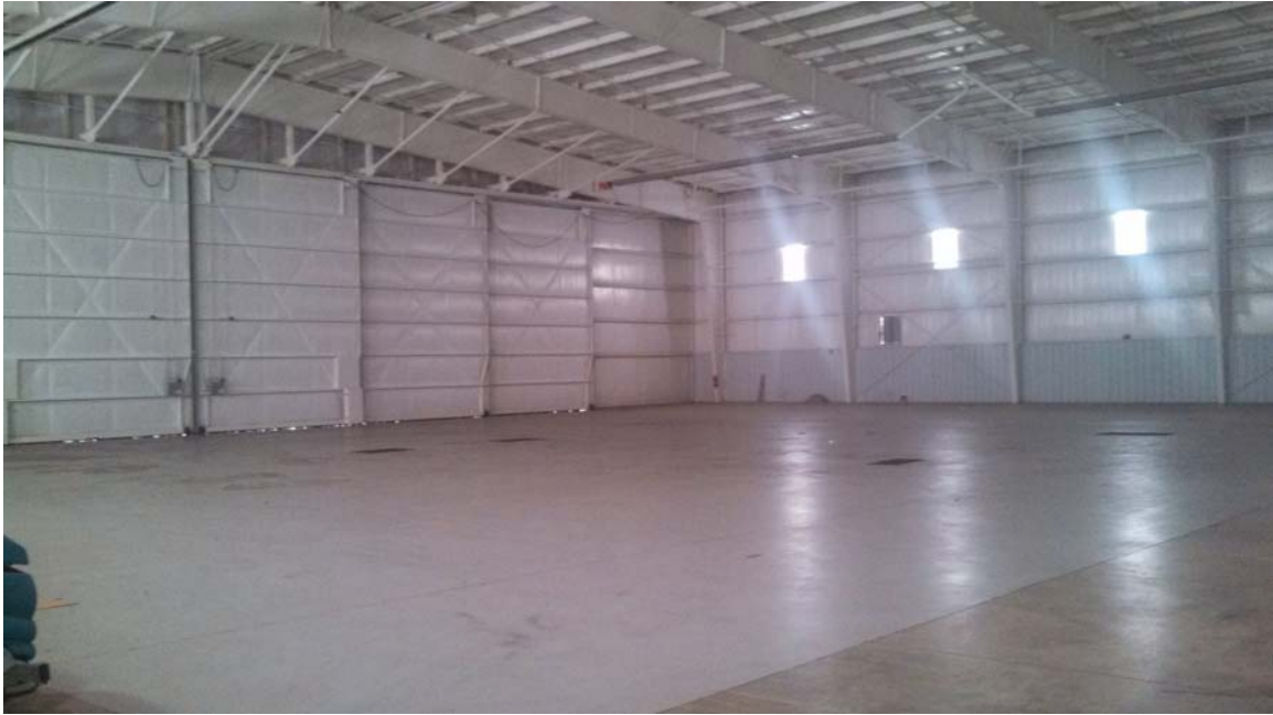
Interior Shot of Hangar
