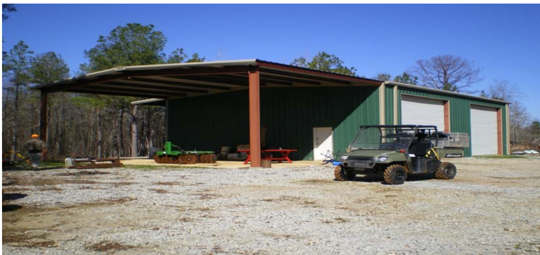
New constructed pole barn – two-thirds enclosed
