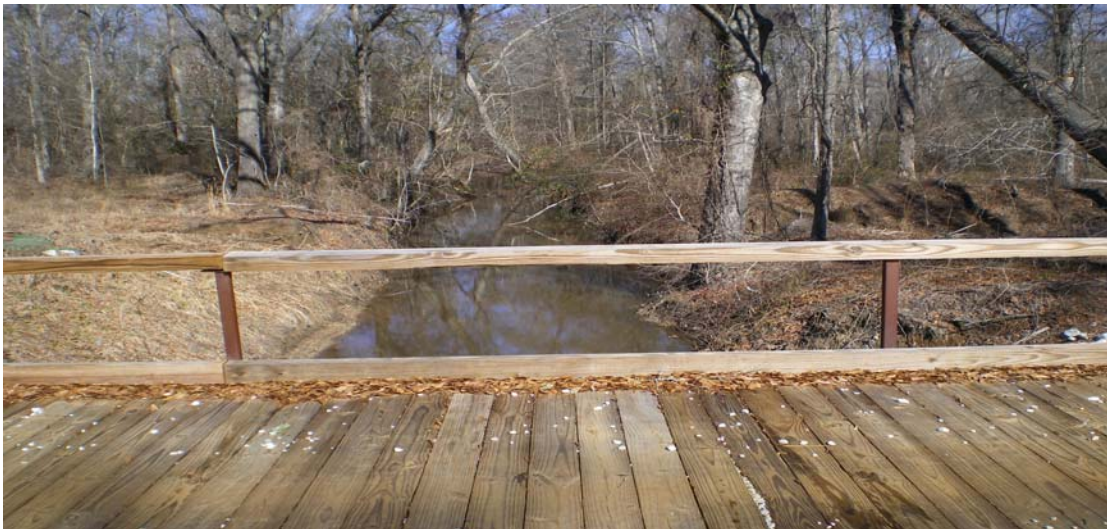
Bridge over the creek
