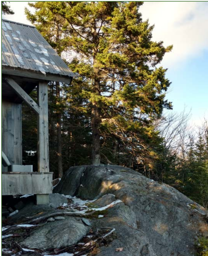
The cabin is built right to the edge of the bedrock. Here, the land falls away and the views are grand.
