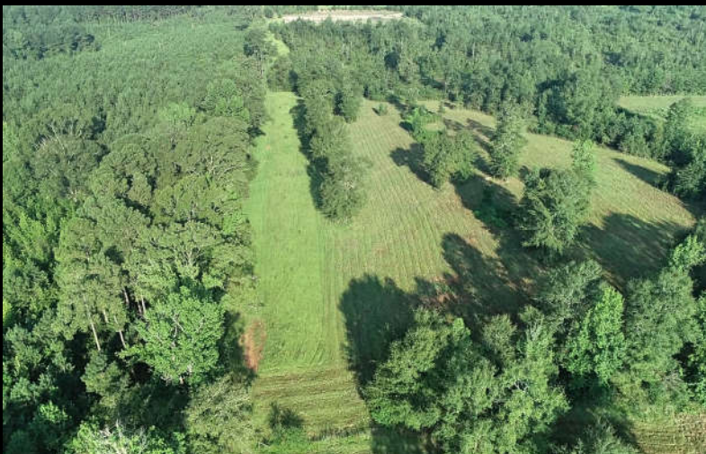
Aerial View of Pipeline
