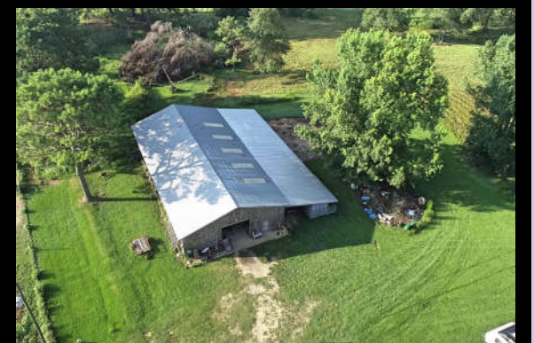
Aerial View of Barn
