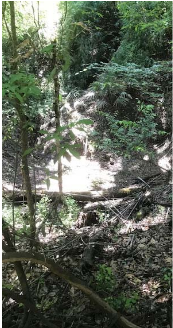
View from bottom of sinkhole areaInterior view
