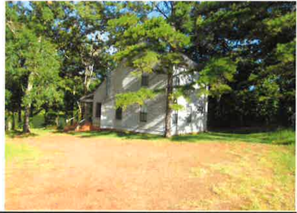
REAR VIEW OF GUEST HOUSE
