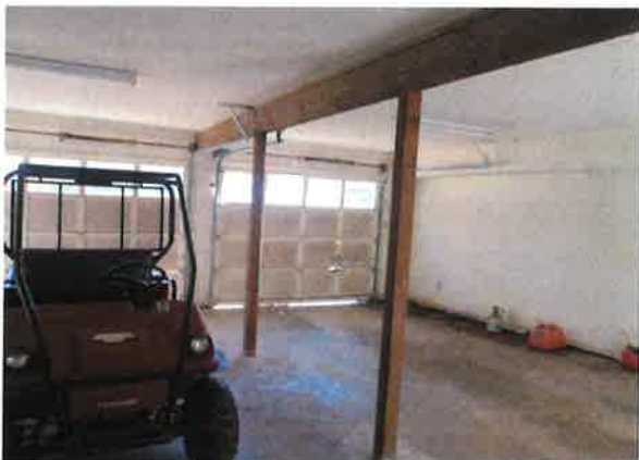
INTERIOR VIEW OF GARAGE AREA - GARAGE APARTMENT
