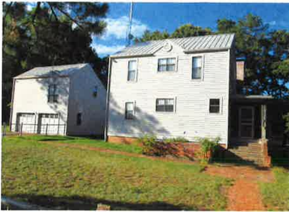
FRONT VIEW OF MAIN RESIDENCE AND GARAGE APARTMENT
