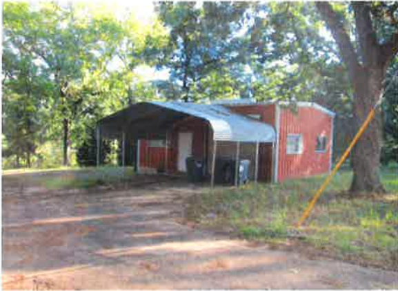
VIEW OF SHOP AND METAL CARPORT
