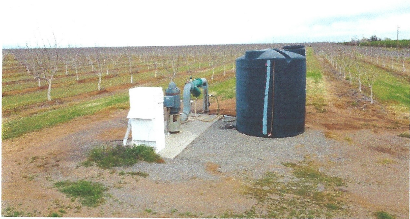
well 16 in. casing 760 Ft. depth
