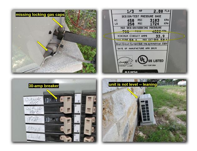
Recommend consultation with Electrical & HVAC contractors to address/repair deficiencies and perform general maintenance on system.
