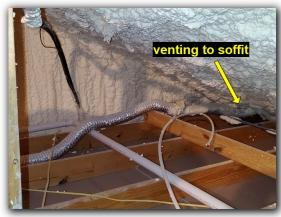
Recommend routing all exhaust fan ducts to the exterior of the structure
