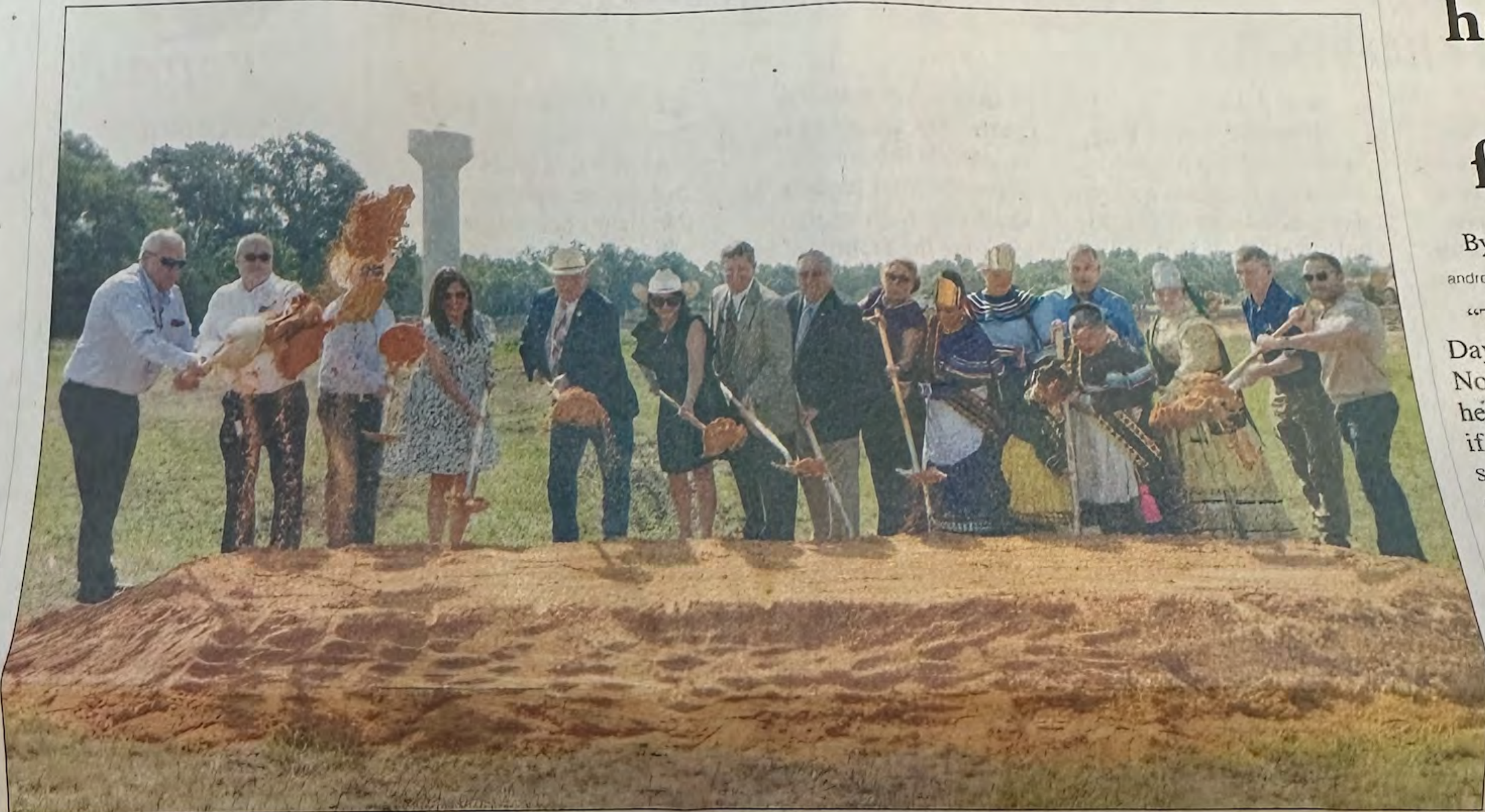
Poarch Creek Indian officials, state officials, Escambia County commissioners and Perdido River Farms employees break ground on the new meat-processing facility May 25.
