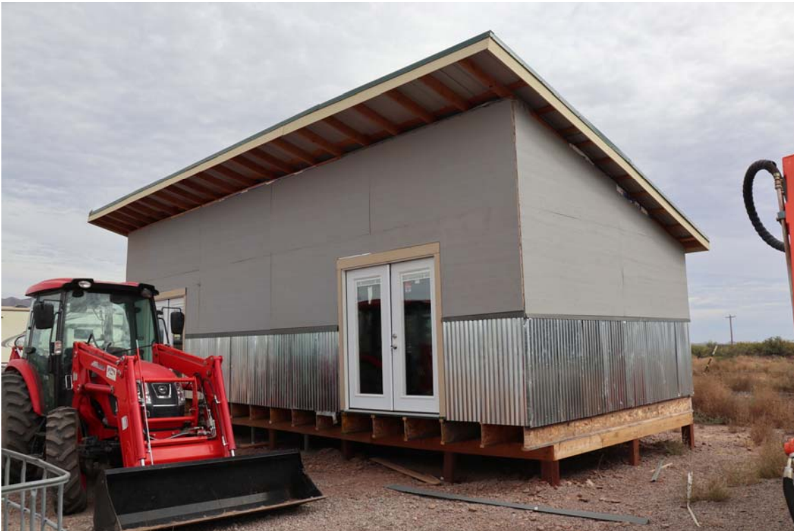
Office/apartment, partially complete
