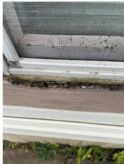
exterior window trim
