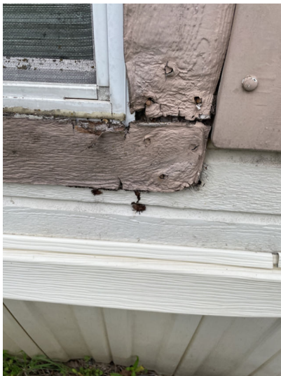
exterior window trim
