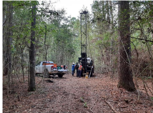
Facing Northwest at Boring B-05
