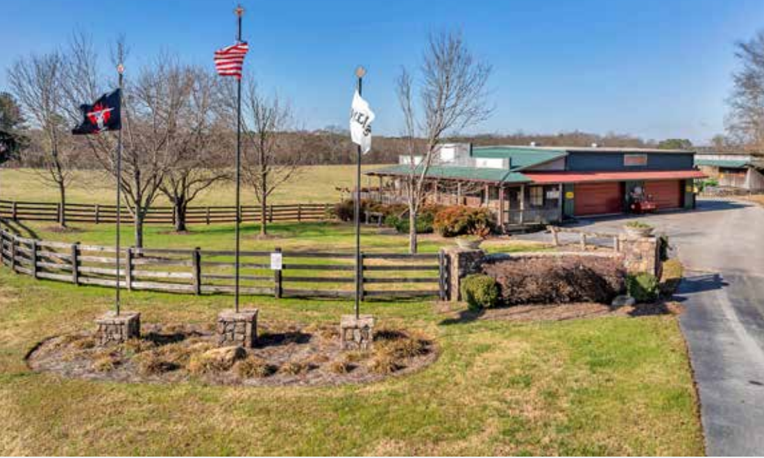
Green Roofed Metal Barn near the Entrance
